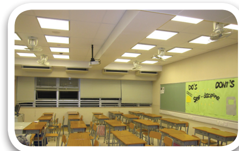
LED panel lighting at classroom 課室內的LED燈盤照明
