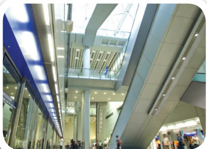
Replacement of fluorescent luminaries and metal halide with LED luminaries at Automated People Mover Platform 將無人駕駛列車月台的螢光燈及金屬鹵化素燈更換為LED燈
