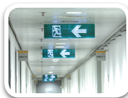
LED exit sign LED 出口指示牌
