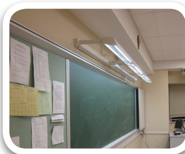
LED tubes for green board lighting at classroom 課室內用作綠板照明的LED光管
