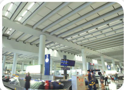
Replacement of fluorescent luminaries with LED luminaries at Baggage Reclaim Hall 將行李認領大堂內的螢光燈更換為LED燈
